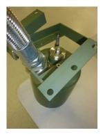
Supply Recirculation Monoline Coaxial Hose Assembly:
